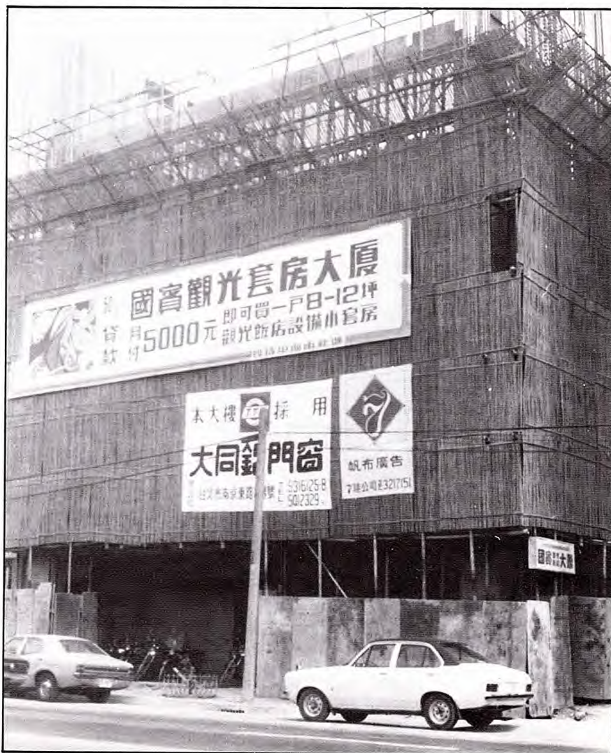
A common sight on Taipei streets is this bamboo scaffolding on a new bank building.
