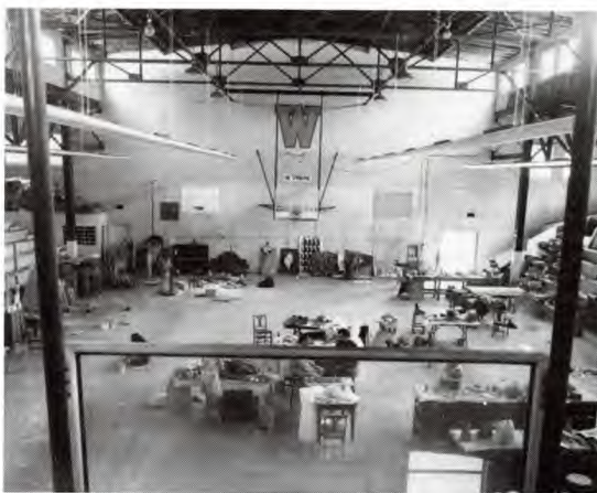
1990: Transformation in progress from Theatre Arts storage/set design to Art Department classrooms and offices.
