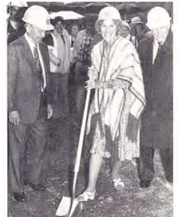
Trustee Charlotte Graham beams as she turns the first shovel of dirt at Groundbreaking.
